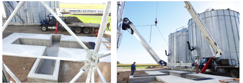
The shallow double drive over is modular by design and can be custom configured to fit your application. It can be installed under truck scales or simply in a shallow trench under a driveway. The shallow design minimizes concrete and dirt work during installation while maximizing efficiency for the operation once installed.
