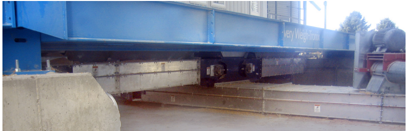
Overview of double drive over installed under Weigh-Tronix scale.
