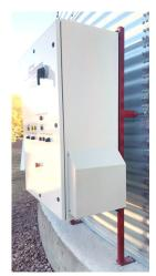
Simple installation: Site electrician supplies incoming power to the panel and connects it to the motor.
